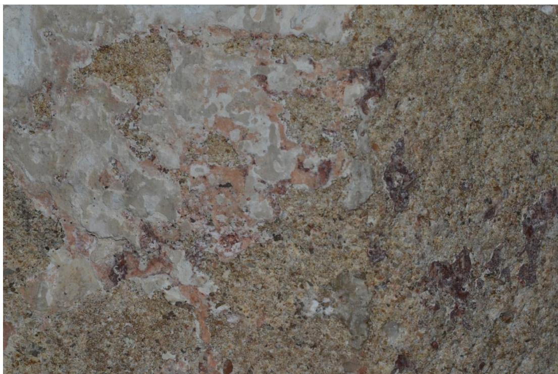
Traces of red and pink paint partially surviving on the SE face of the western pier of the south arcade. The paint can be seen to be overlain by one or two coats of limewash with dirty (grey) surfaces.
