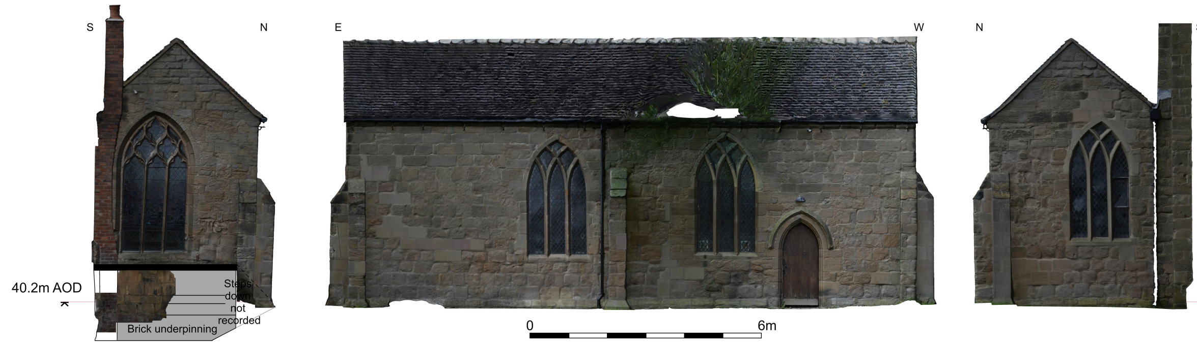
Exterior elevations of north aisle. L-R: East face of east wall looking west, with boiler room below; north face of north wall looking south; and west face of west wall looking east.
