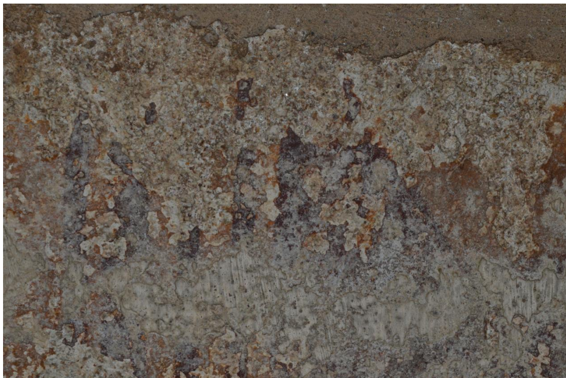
Traces of red and yellow paint in the eastern splay of the squint in the south aisle showing overlying limewash layer with dirty surface.
