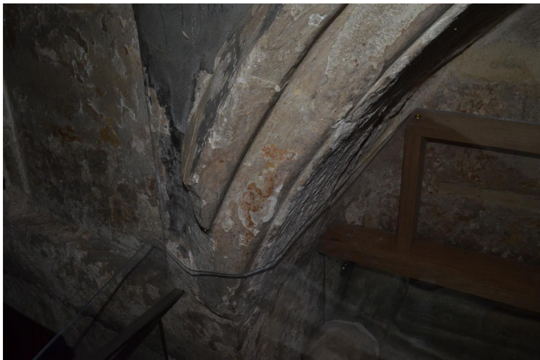
Yellow paint on the moulding on the eastern side of the tomb recess in the south wall of the south aisle. Photo looking south east.
