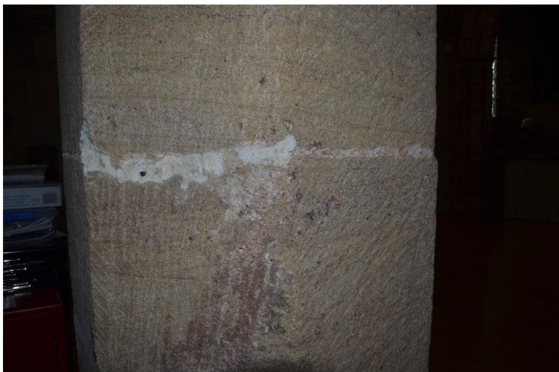
Traces of pink and red paint surviving on the heavily stripped SE and E faces of the western pier of the south arcade. Photo looking north west. See below for detail.
