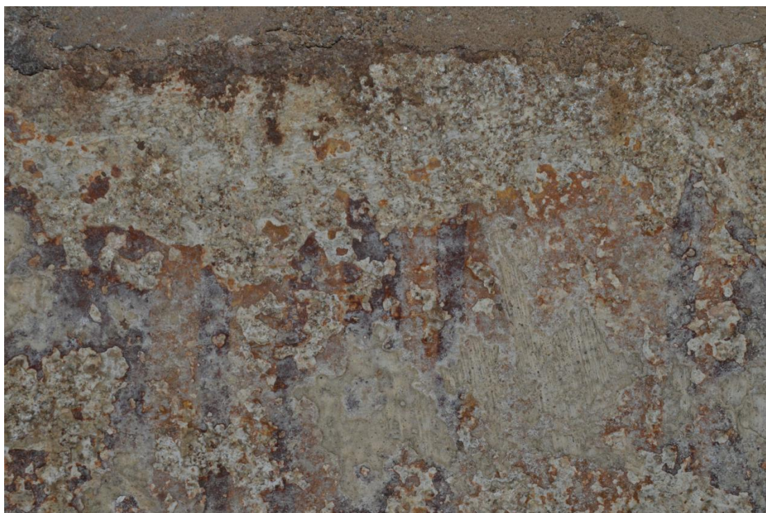
Decoration on the eastern splay of the squint in the south aisle, showing yellow ground with broadly parallel curving vertical red lines, partially obscured by limewash with dirty surface. This stone located immediately beneath that with the horizontal lines above. Photo looking north east.
