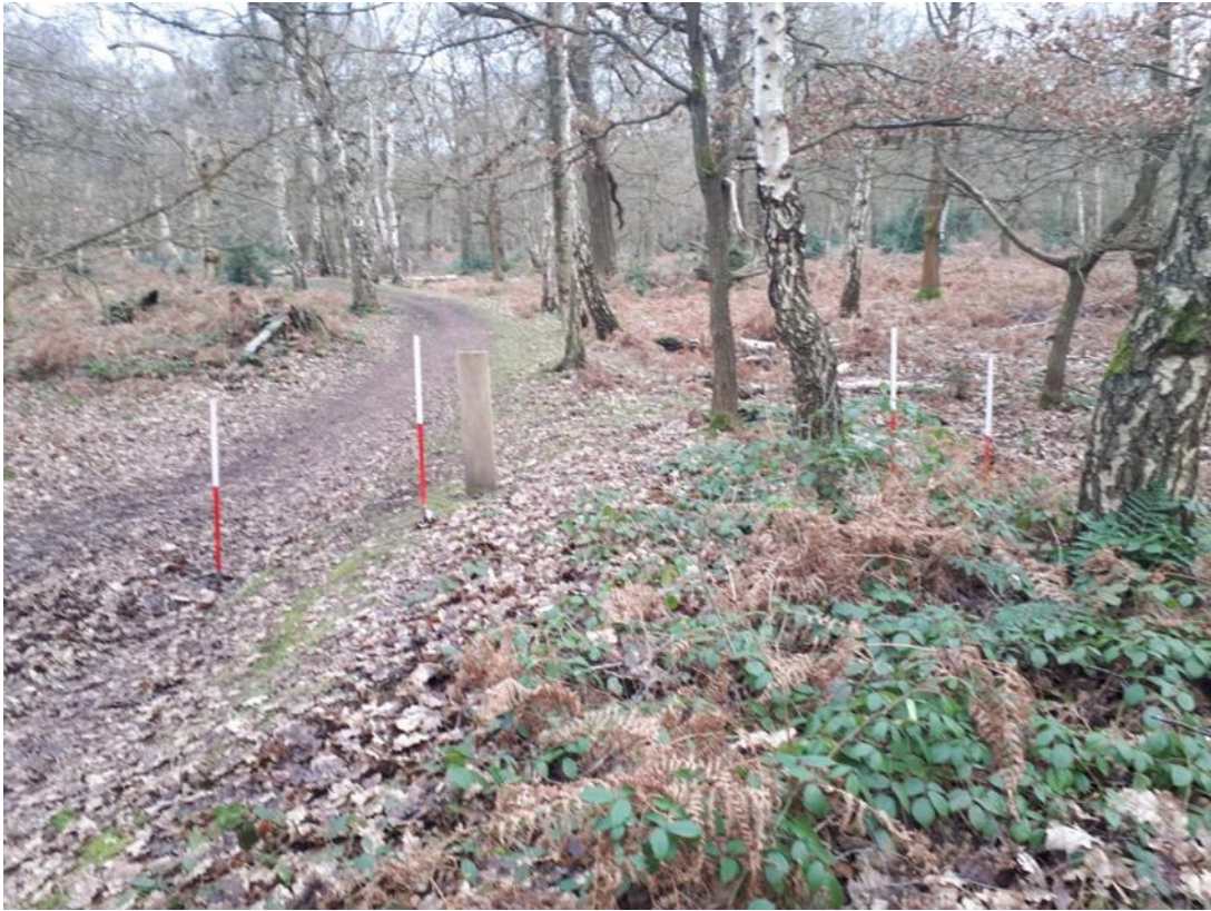
Photograph A_9 : Railway embankment in Birklands Wood.
