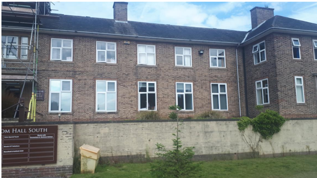
Photograph M_1: Ransom Hall, former Hospital. The basements are situated under the building shown,
