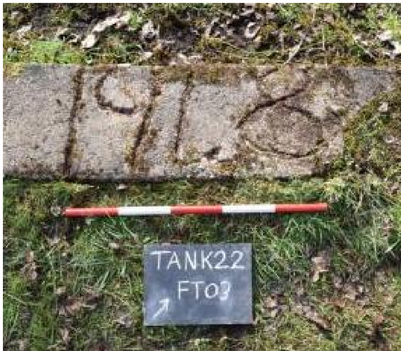
Photograph N_5: Close up of Cill. When decommissioned as an Immersion Tank, the system was converted into a swimming pool and used by local children. Concrete cills were added at the top of the
