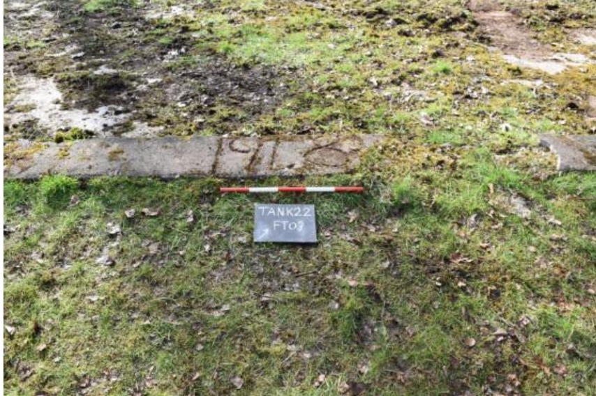
Photograph N_4: When decommissioned as an Immersion Tank, the system was converted into a swimming pool and used by local children. Concrete cills were added at the top of the two ramps into the chamber to prevent dirt and debris washing in and to retain the water in the pool at a higher level. These cill across the Eastern side has the year 1948 scratched into the cement while still wet, providing a Terminus Ante Quem for the use of the feature by the military.
