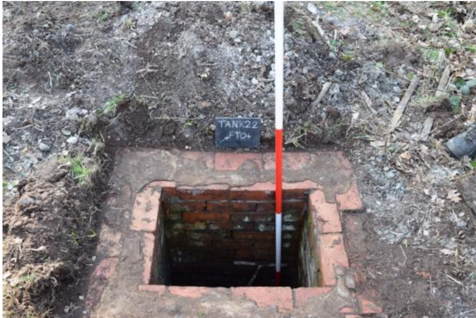
Photograph N_8: Brick-lined access chamber- south of inlet on exterior side of wall.
