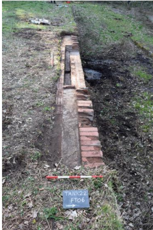
Photograph N_2: Overflow system. Southern wall of Immersion tank. Cleared to show construction. Header Bricks act as capping to the double brick this interior wall on the left of the picture. A 35cm thick fill of concrete is then lined with a single skin of bricks on the exterior side. A mortared channel drains into a grate in the centre. Photo facing West.
