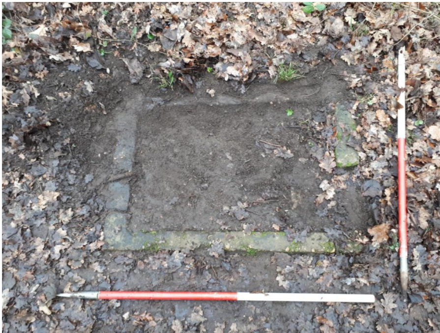
Photograph E_5: Concrete feature- probably remains of part of a building, dating from WWII. In the former POW and displaced persons camp, Edwinstowe.
