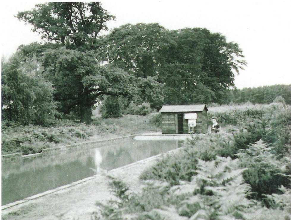
Figure N_15: The Tank wash converted to a swimming pool complete with newly constructed changing hut on the western end. Photo facing South-west.
