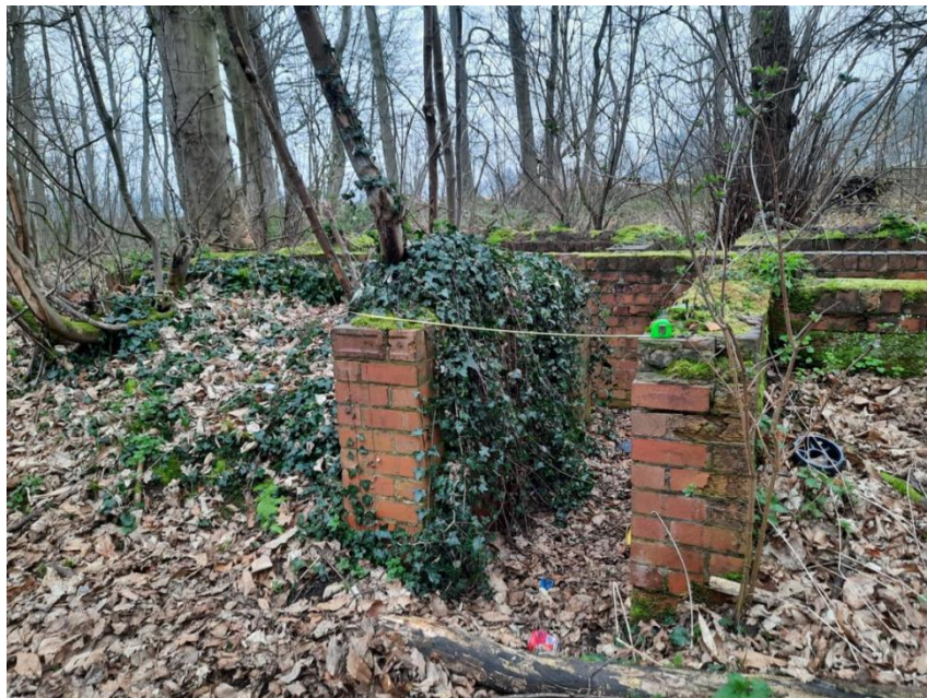
Photograph L_3: Brick Hut remains
