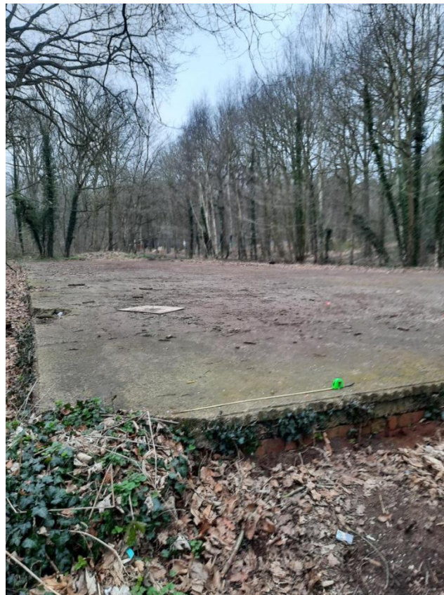
Photograph L_1: Concrete building platform.
