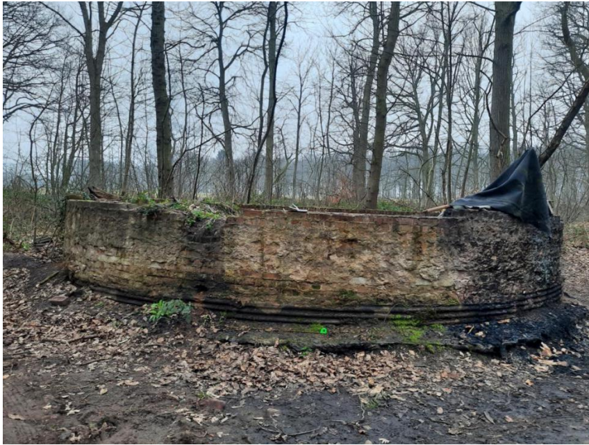
Photograph L_2: Circular concrete structure.
