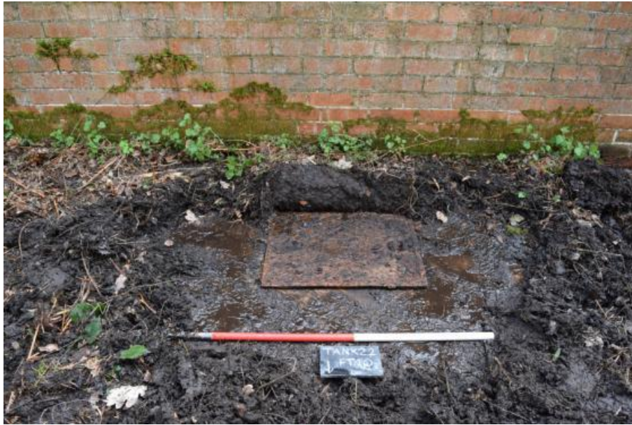
Photograph N_6: Iron Manhole cover for draining the system. Located in the centre of the system east to west, on the southern side of the chamber.
