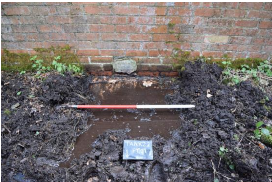
Photograph N_7 Blocked-up (mortared) inlet hole in southern wall of chamber
