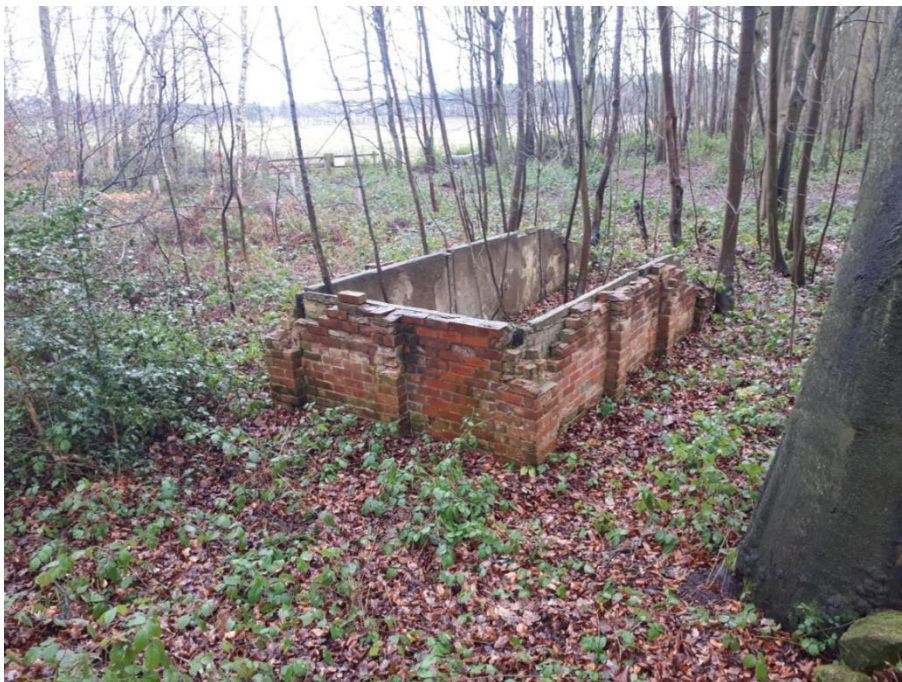
Photograph J_2: Remains of a brick military building, internally rendered in mortar, in proximity to the railway platform above in photograph J_1. In Thoresby North Woods, former ammunitions store.
