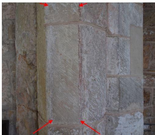
Plate 59 - southern side of chancel arch, at position C3 and C4 of Figure 01, showing medieval paint and limewash layers stopping at vertical lines indicating position of original screen (between the arrows). Looking south, direct flash.
