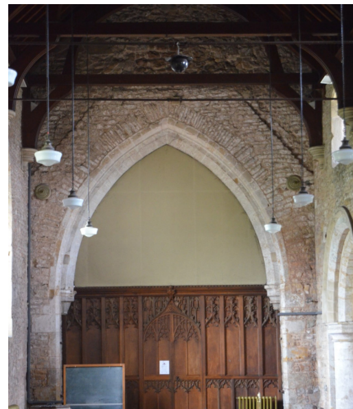
Plate 10 - scars of former roof lines on east facing wall of tower (dark diagonal lines above the (later) tower arch). Looking west.
