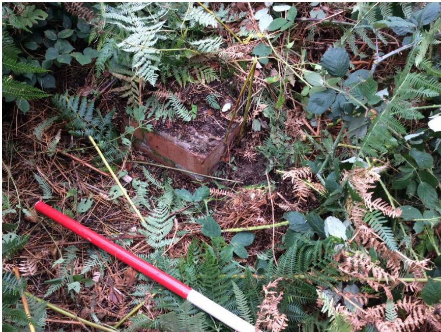
Photograph 12: CARB18006: Hut Platform, brick lined concrete base. Facing north.
