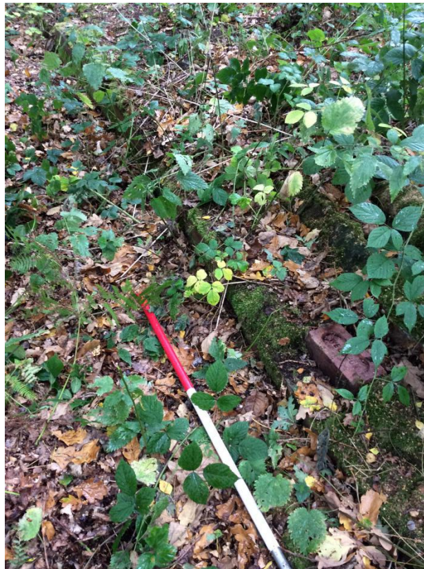
Photograph 02: CARB18001: Hut Platform, brick lined concrete base. Showing 'Welbeck' brick used in construction. Facing west-north-west.
