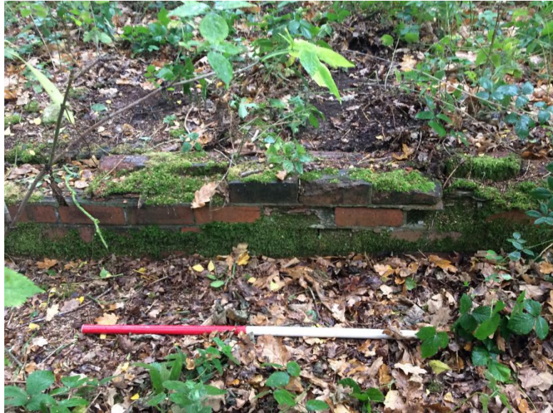
Photograph 03: CARB18002: Hut Platform, brick lined concrete base. Showing 'Welbeck' brick used in construction. Facing north.
