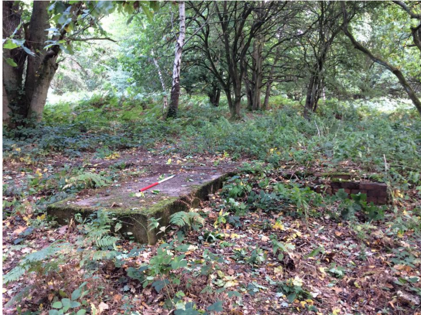
Photograph 05: CARB18003: Hut Platform, brick lined concrete base, with projecting extension on western end. Facing north-east.
