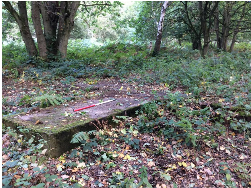
Photograph 06: CARB18003: Hut Platform, brick lined concrete base, with projecting extension on western end. Facing north-north-east.
