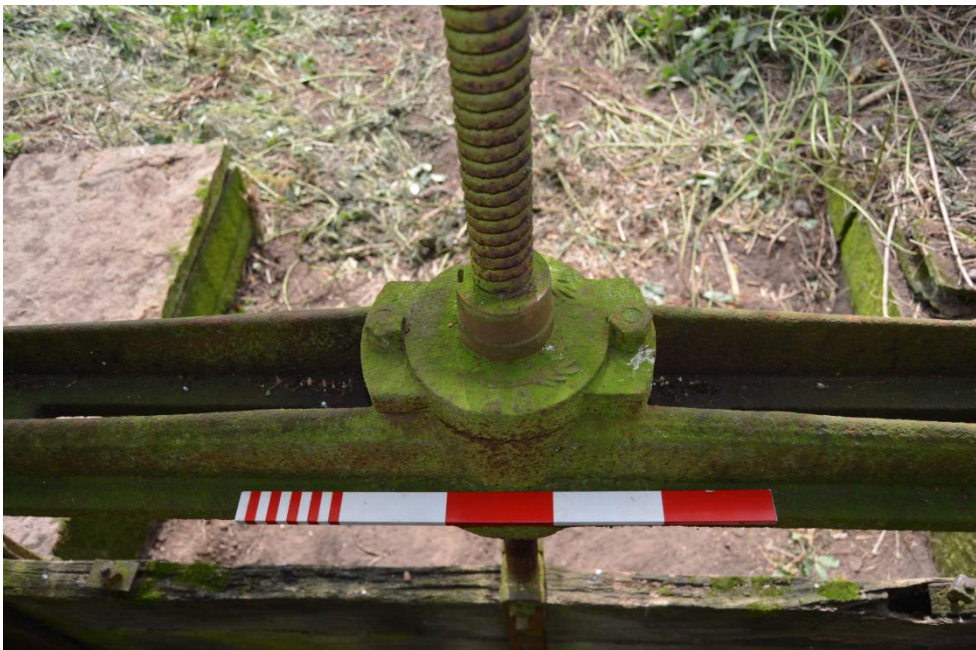
Photograph: Iron winding screw for opening wooden sluice gate CUCK18WM009, facing west.
