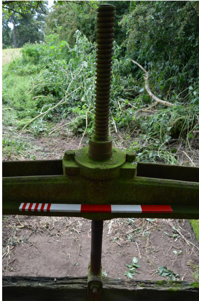
Photograph: Iron winding screw for opening wooden sluice gate CUCK18WM009, facing west.
