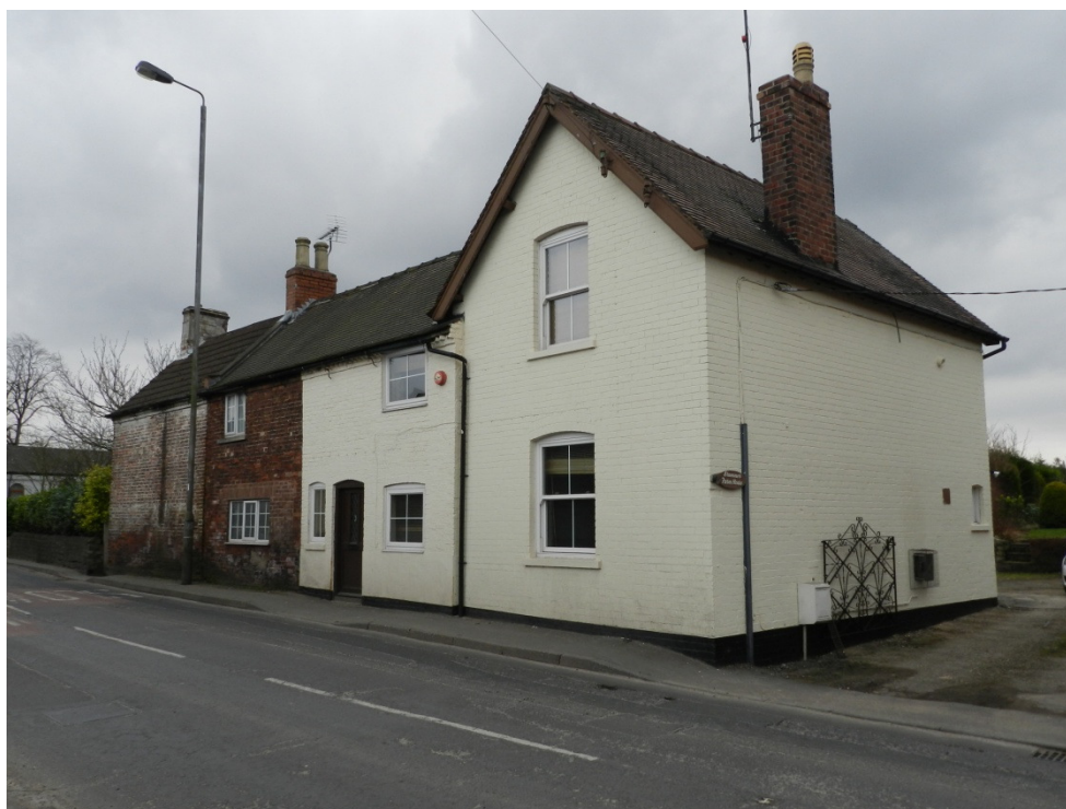
Fig 25 The site, looking south-east
