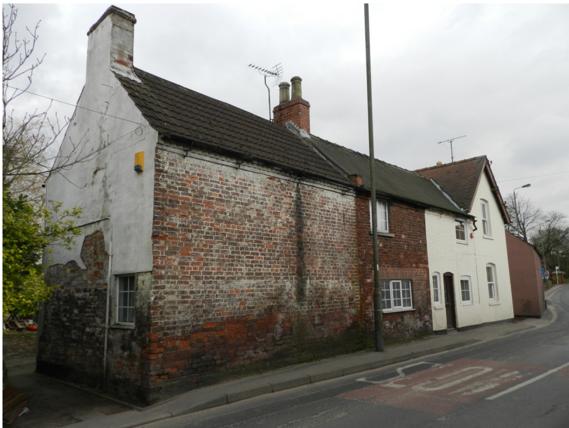
Fig 22 The site, looking south-west
