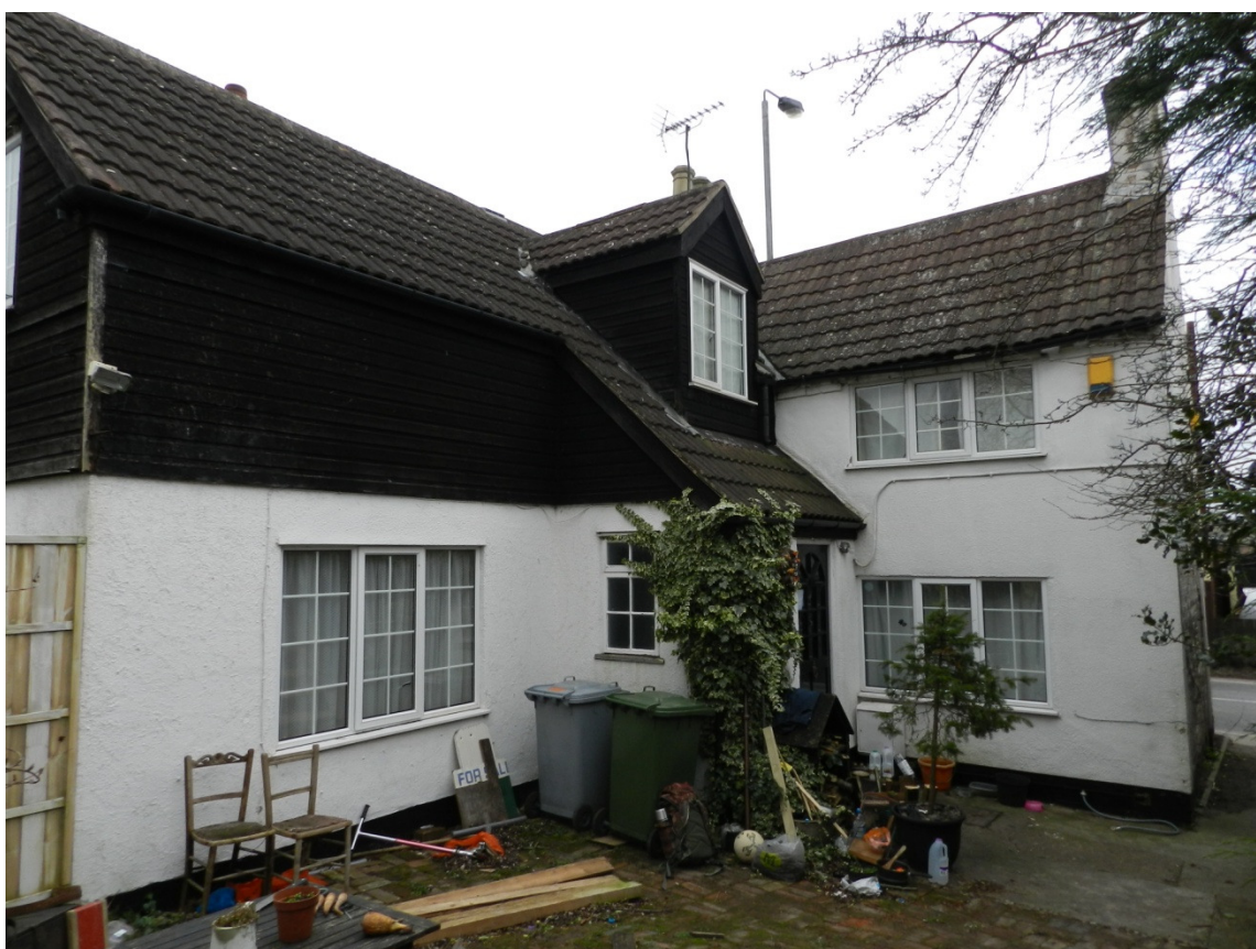
Fig 23 The south and east elevations of Arundel Cottage, looking north-west
