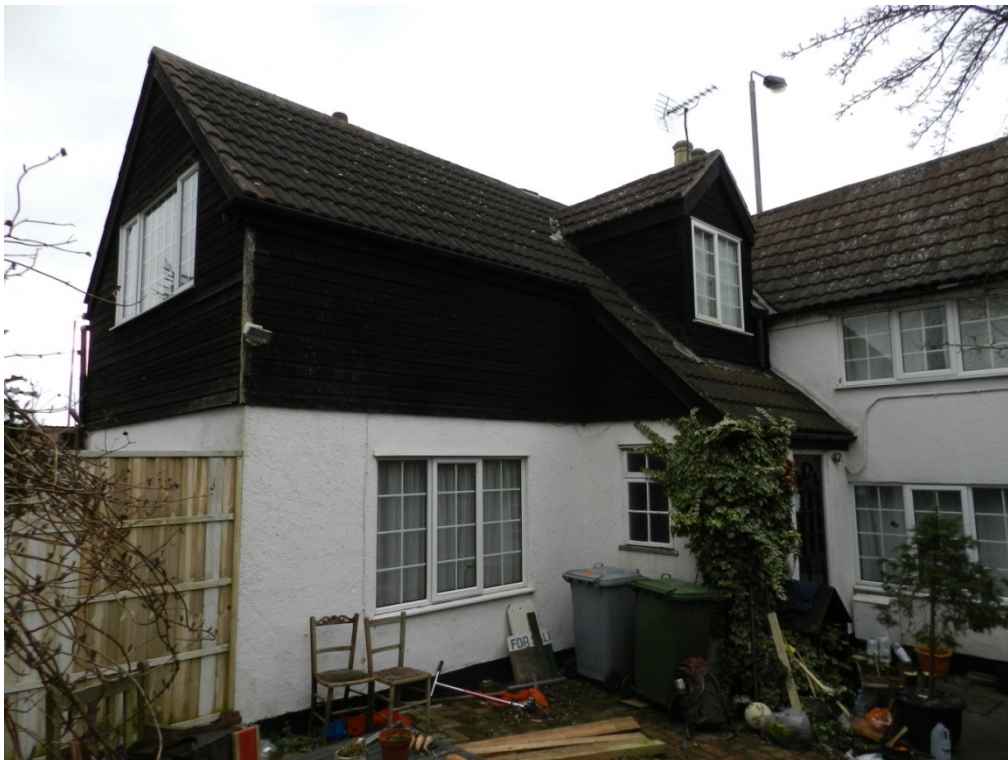
Fig 28 The extension to the south of Arundel Cottage, looking north-west
