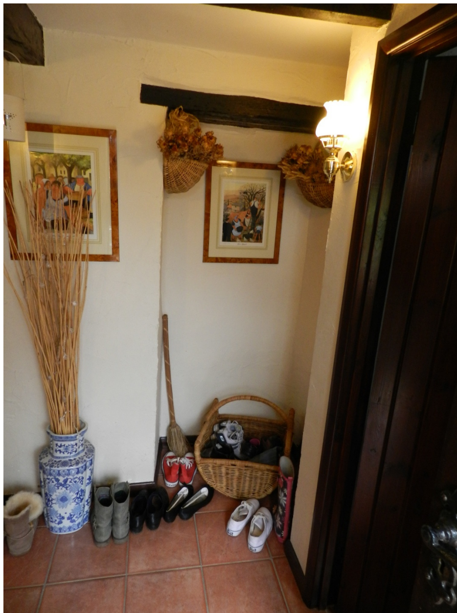
Fig 13 Blocked splayed opening in Stone Wall 2, looking north
