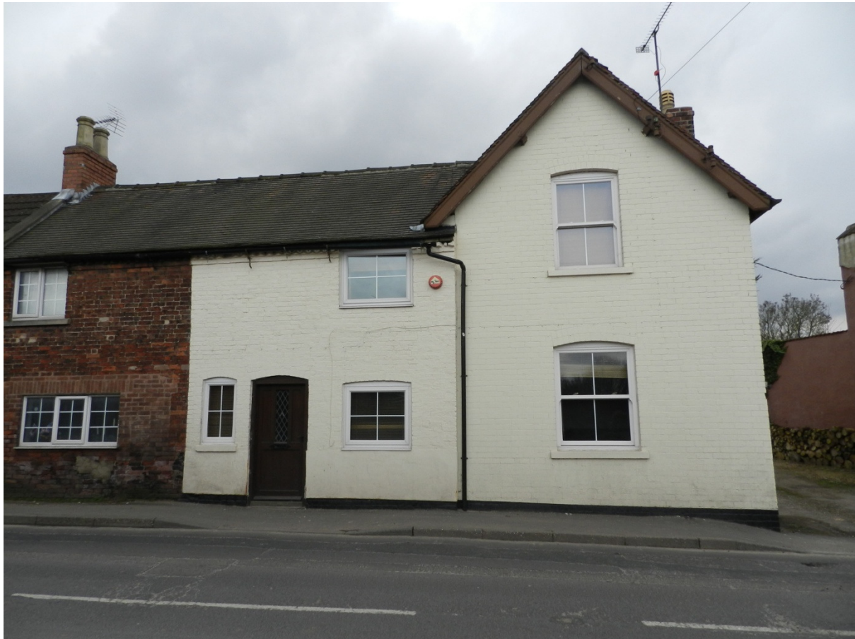
Fig 15 The north elevation of Brammer Farmhouse, looking south
